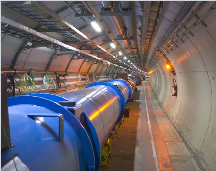
Blick in den Tunnel
